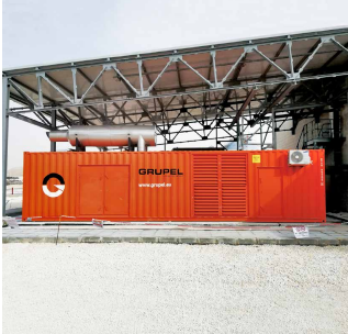
Installation in Jordan
