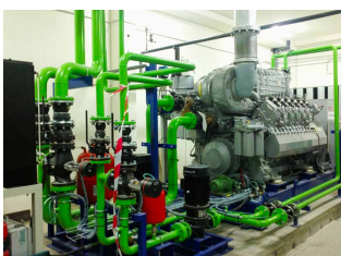
Installation in Spain
